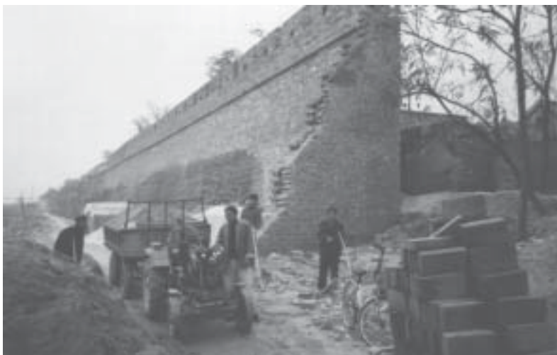
Shangqiu city wall undergoing reconstruction, November 2002
